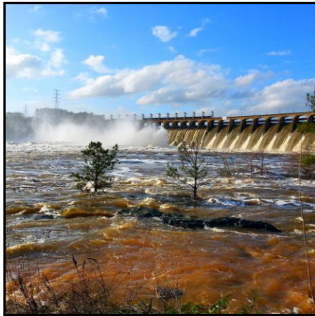
Lake Jordan Dam flooding after heavy rains
